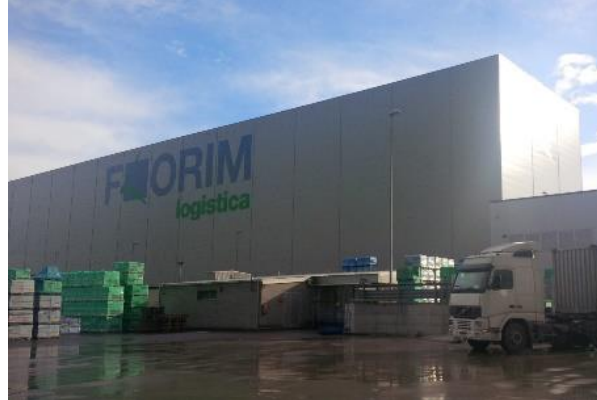
Central DC @ Fiorano Modenese (MO)
